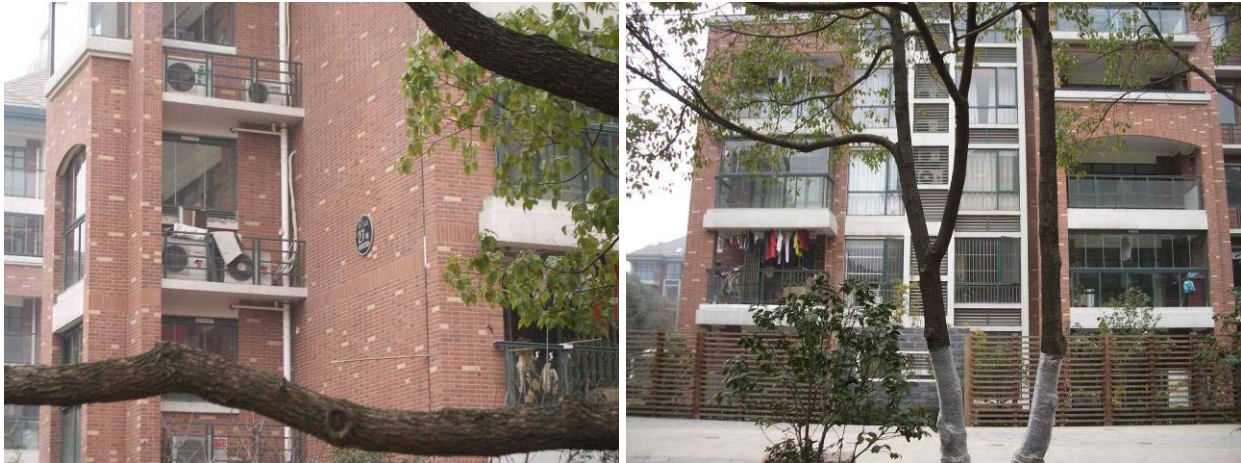
Residential building in Hefei 2007 – decentral heating and cooling for each room
